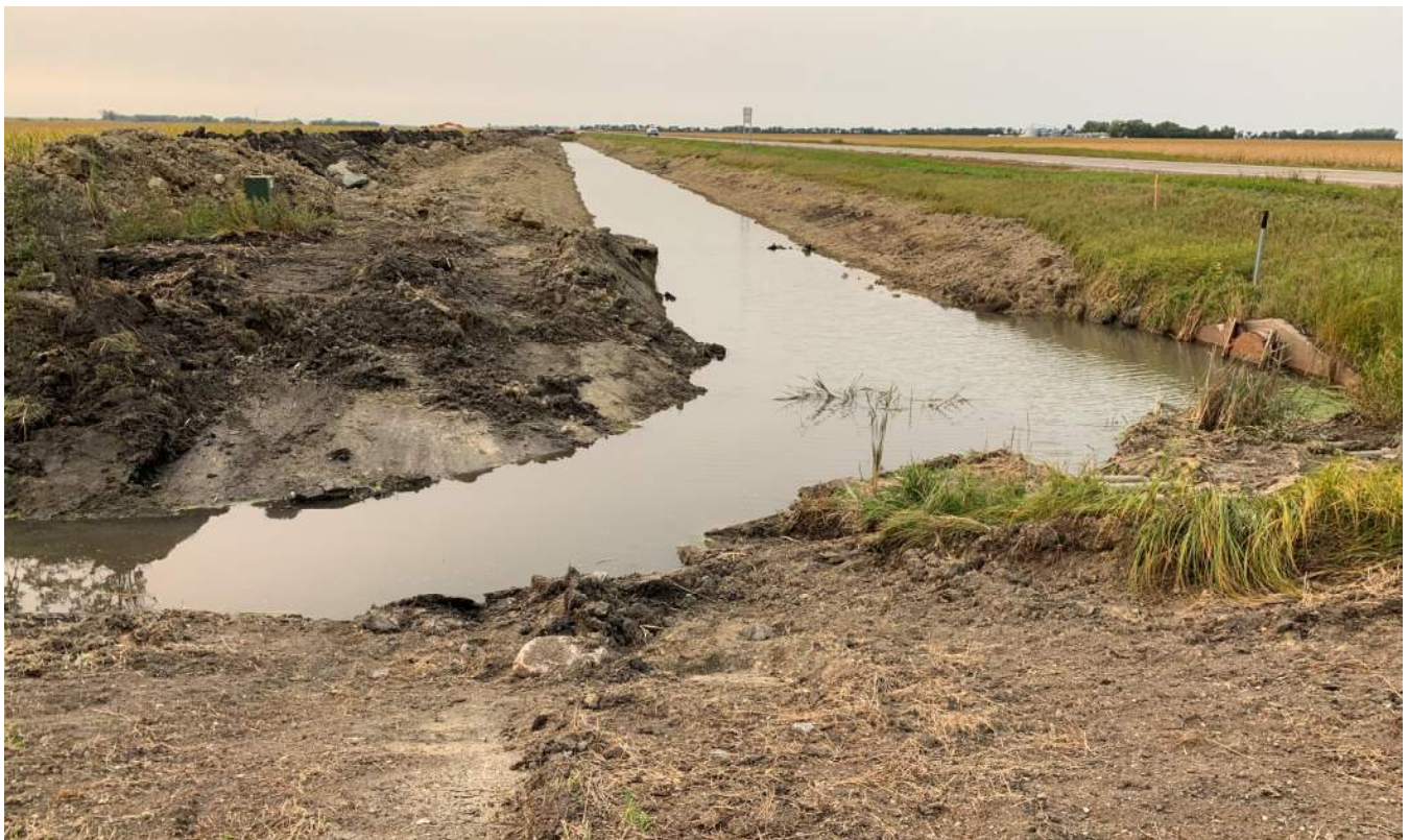
Figure 8: NS Main Section 17 – Excavation (looking south)
