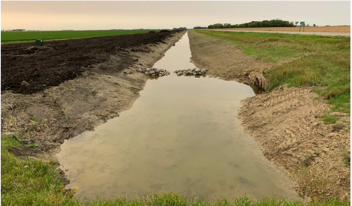
Figure 5: NS Main Section 5 – Topsoil Stripping & Spreading (looking south)
