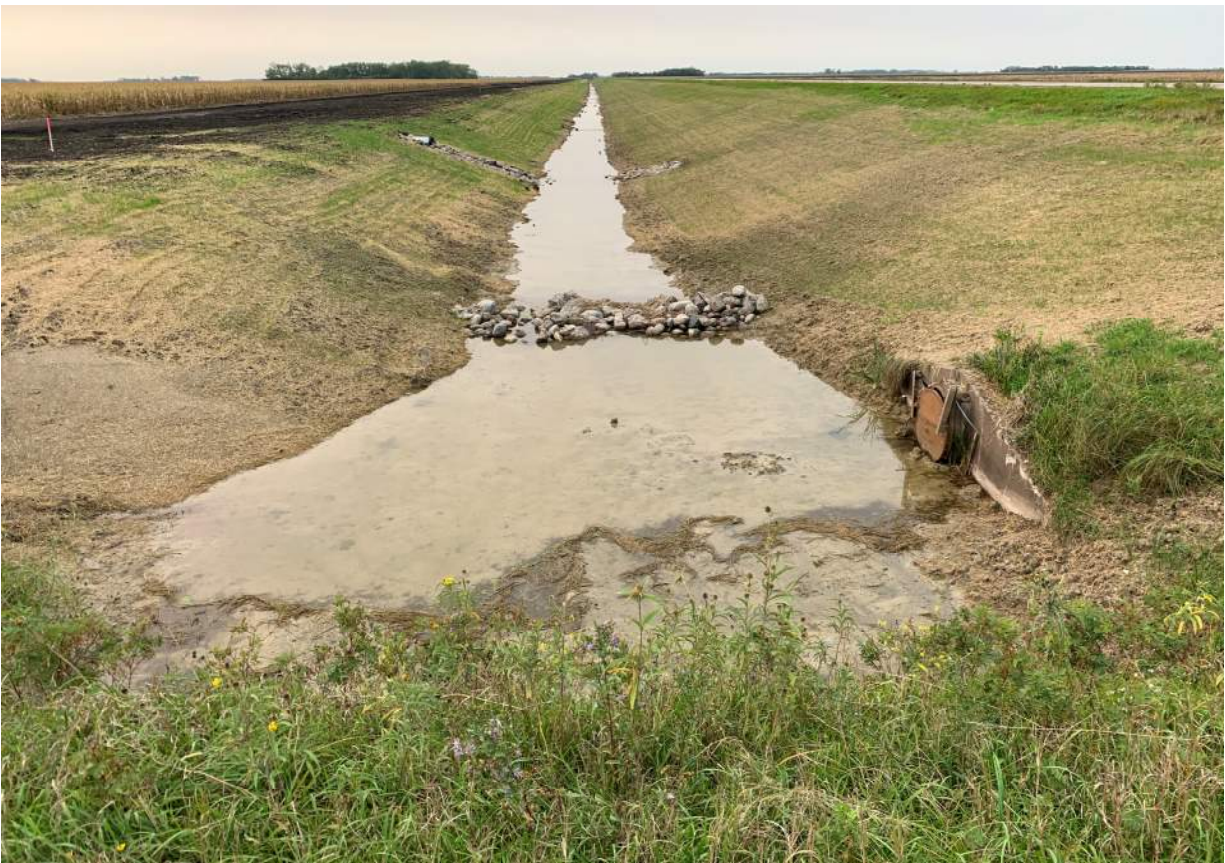
Figure 4: NS Main Section 32 – Seeding (looking south)
