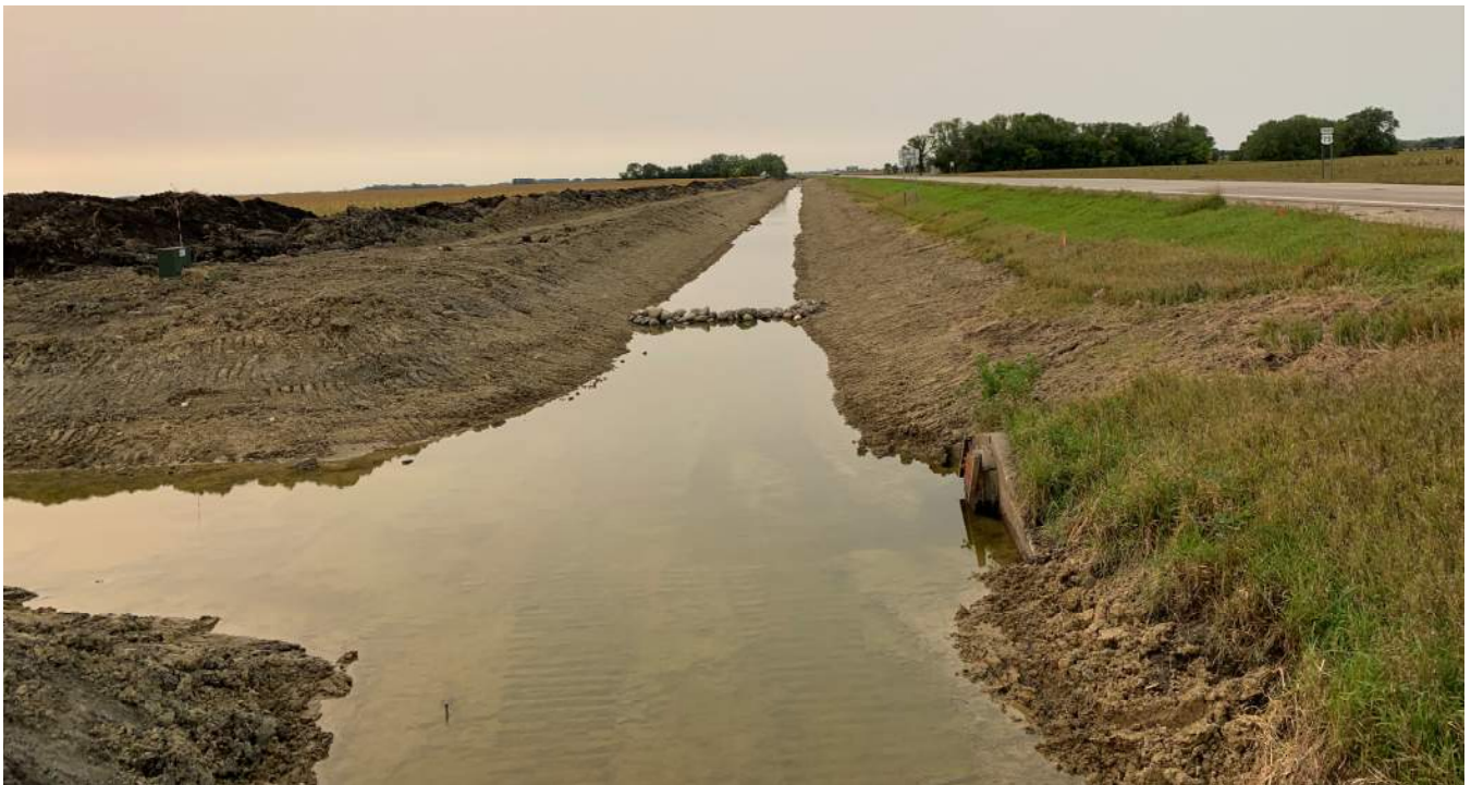
Figure 6: NS Main Section 8 – Excavation (looking south)
