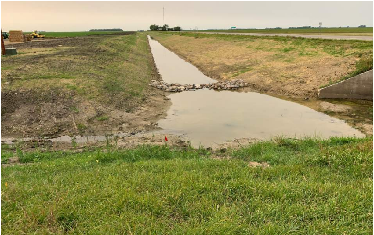
Figure 3: NS Main Section 29 – Seeding (looking south)
