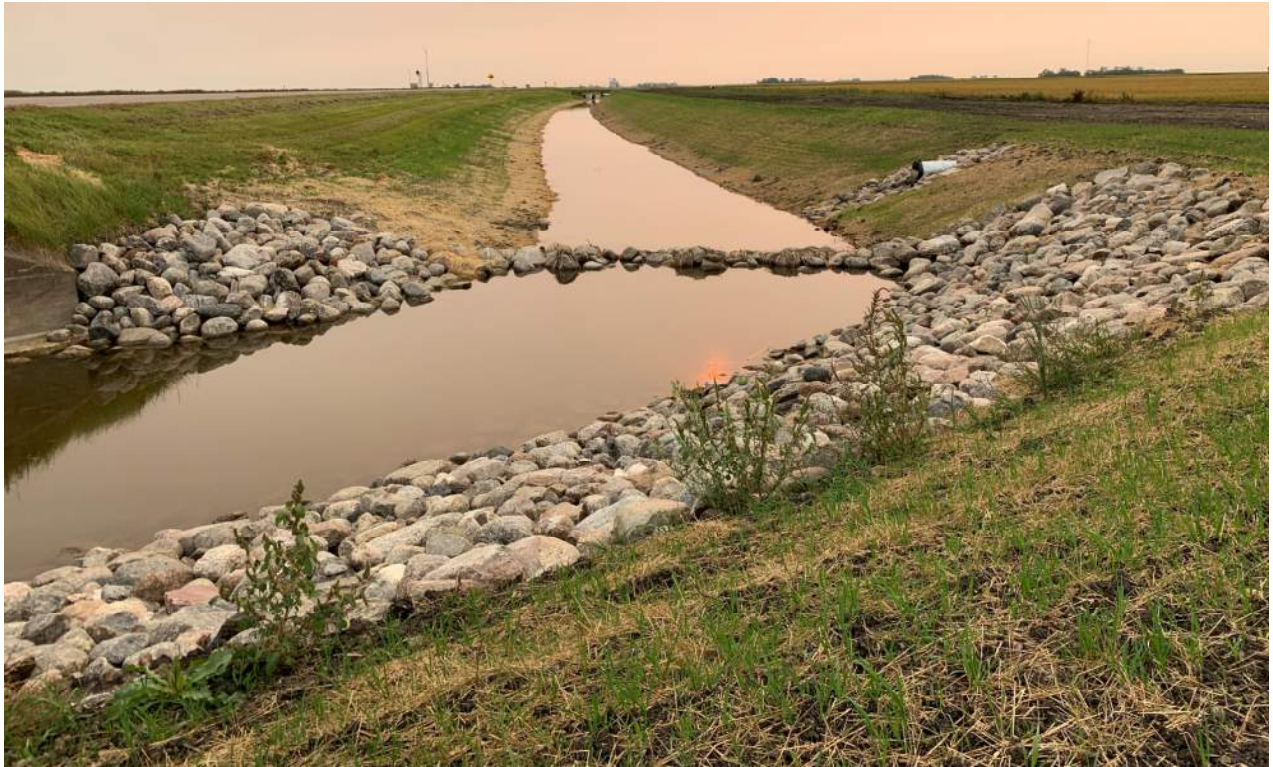
Figure 1: EW Main Section 25 – Seeding (looking east)
