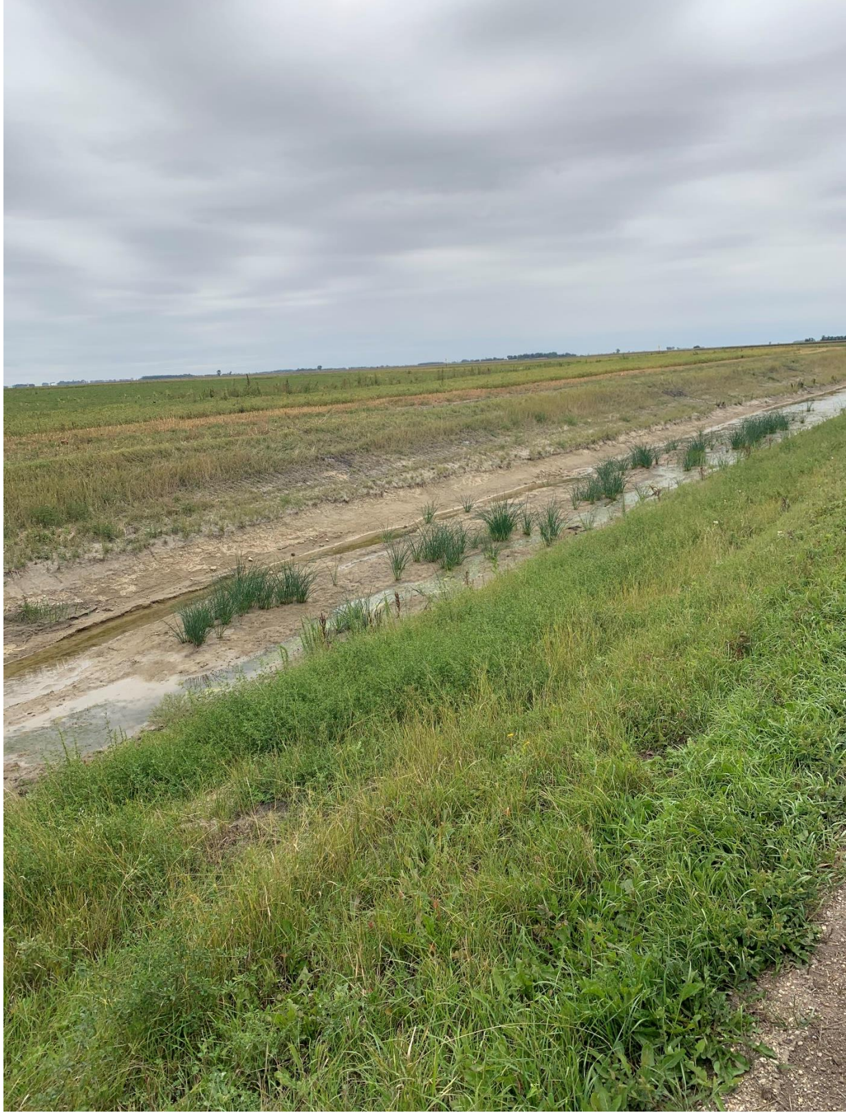
Figure 2: Area along WCD 9 requiring silt removal. 9/11/20
