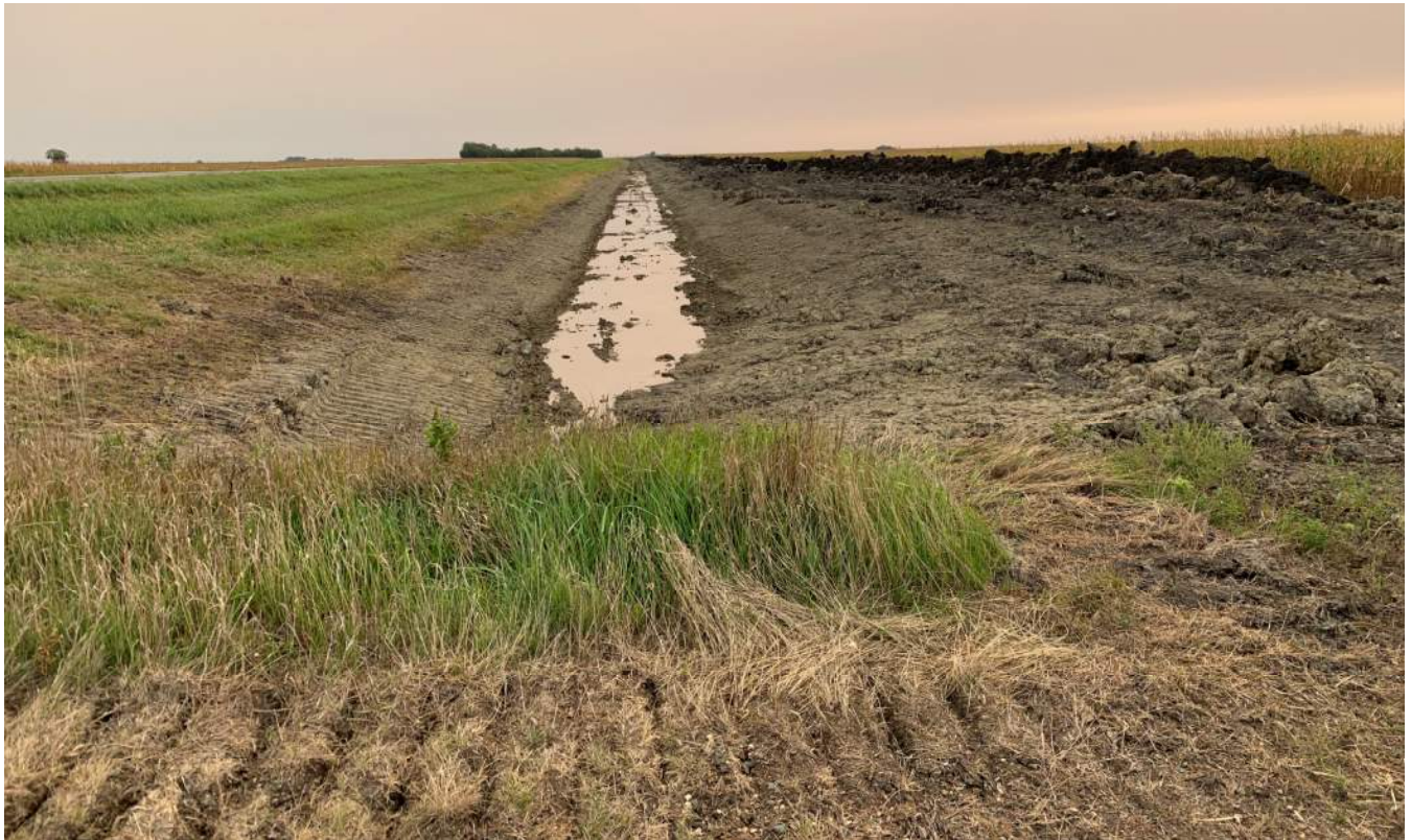
Figure 7: Lateral 6 Section 8 – Excavation (looking east)
